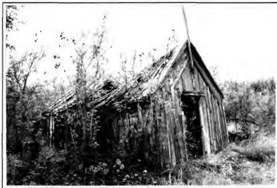
Figure 158. The Miscovich Blacksmith Shop, 1993. The view is looking southwest.
